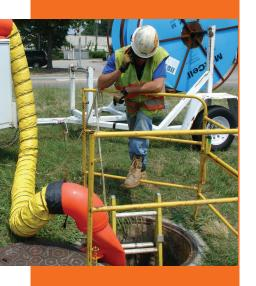
Rugged, Light Weight, Economical Axial Fans to Provide Fresh Air for Confined Space Ventilation
